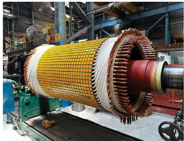
Marthinussen & Coutts restored the 15 MW motor to its original high standards.
