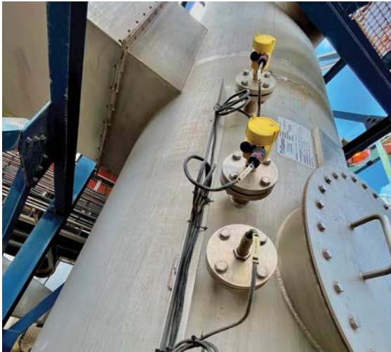
The VEGASWING series of vibrating level switches provides reliable point level detection in a wide range of liquid applications within the energy sector.
