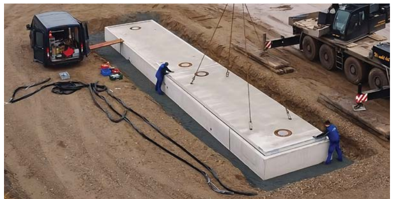
Waagen Dammaschke produces its own precast concrete elements for its truck weighing systems in a wide range of dimensions.
