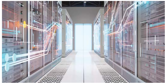
Hitachi and Hitachi Energy support the 800 Vdc power architecture Nvidia is working towards for the next generation of AI infrastructure.
