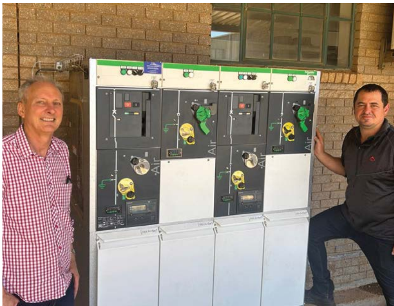
Henk Ryke and Raymond Bosch of TAD with the RM AirSet switchgear.
