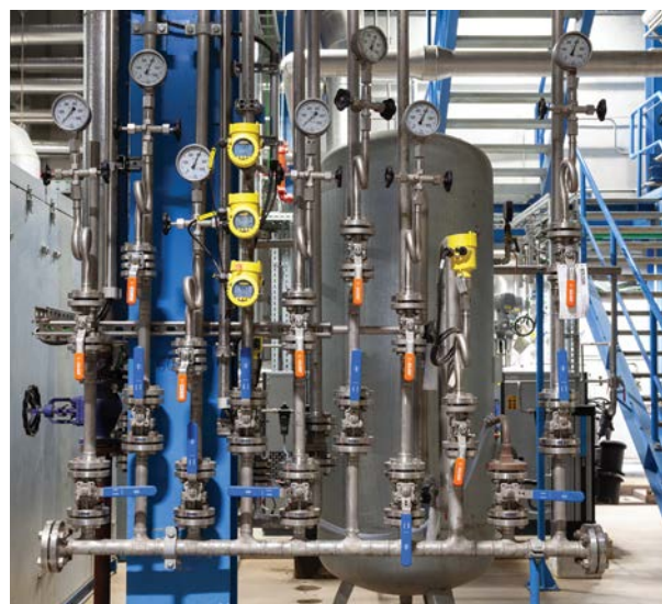
Left: The VEGABAR series of electronic differential pressure measurement sensors. Right: VEGABAR electronic differential pressure measurement sensors here provide steam and condensate process pressure measurement in a paper mill.
