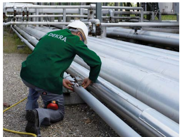
Dekra Industrial offers its customers a holistic service, from non-destructive testing and inspection to industry training.
