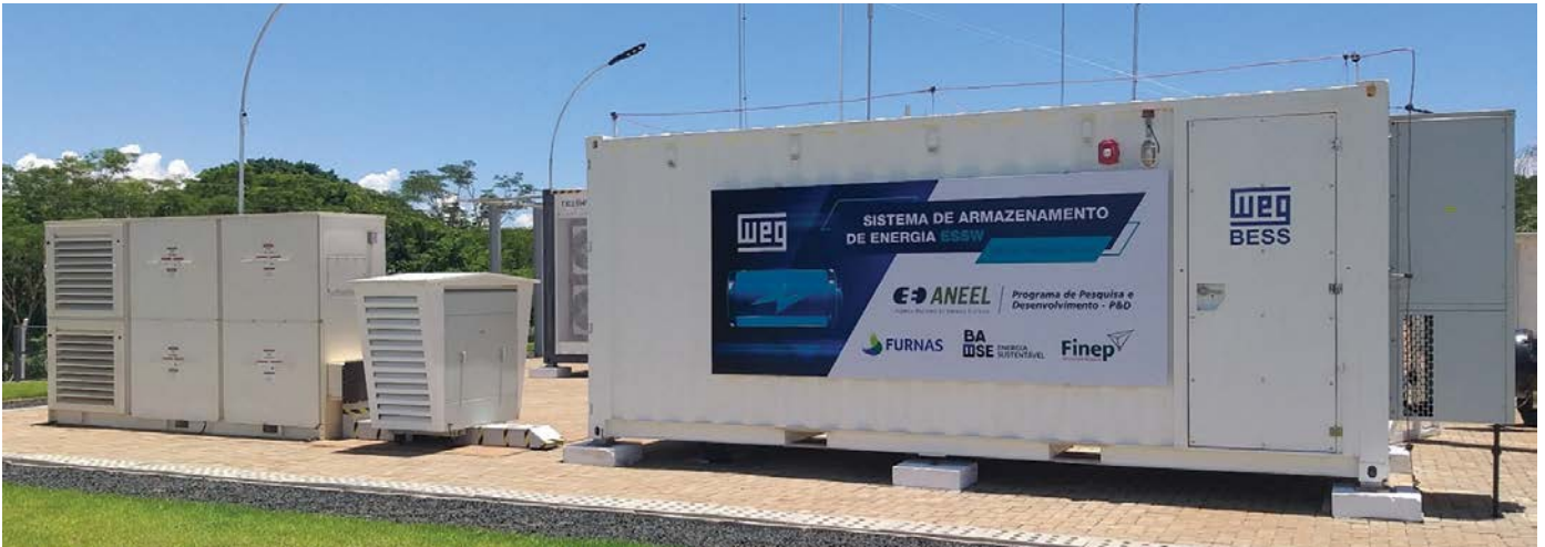
WEG BESS providing support to the first Brazilian H 2 plant (300 kW/600 kWh).
