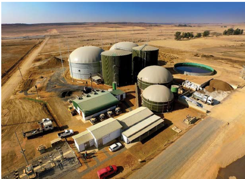
The first Bio2Watt organic biogas plant operating in Bronkhorstspuit, Gauteng.
