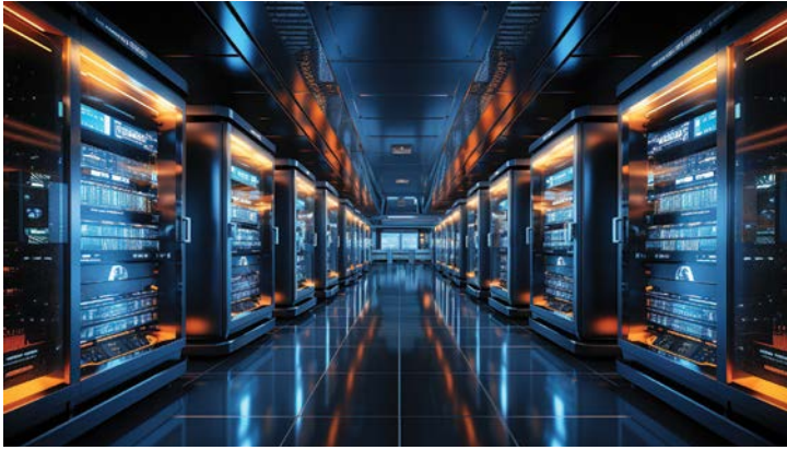
Substation virtualisation will result in significantly reduced hardware needs, with tasks being carried out on cloud servers instead.
