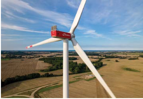
As well as producing the turbine towers for three new wind farms in the Eastern Cape, NESA will supply 57 Nordex WTG Delta4000 series turbines to the project.
