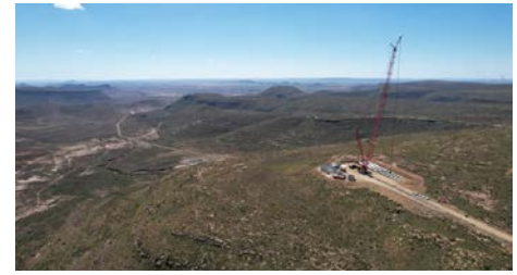
Erecting one of the wind turbines on the site of Koruson 1.
