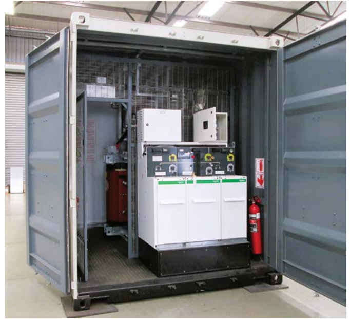
A modular substation in production, being fitted with switchgear for a data centre application.
