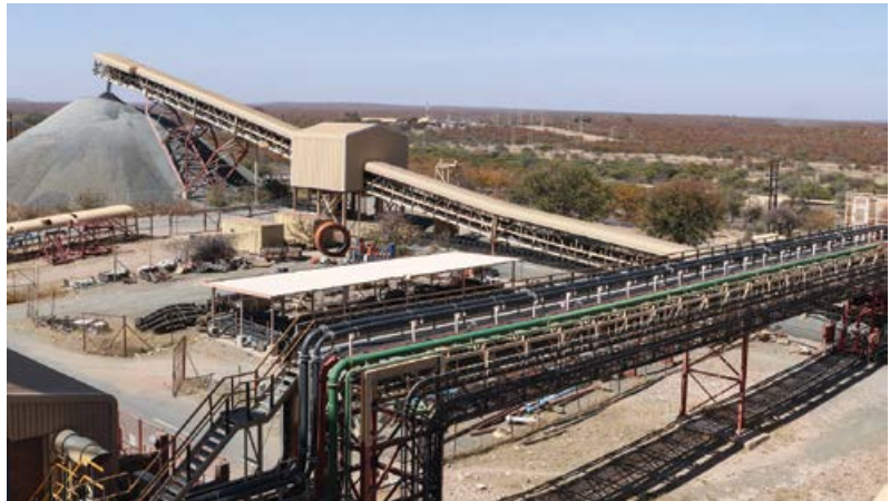
Venetia Mine processing plant.
