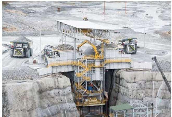
Its wide range of offerings allows FLSmidth to integrate its equipment into an entire semi-mobile in-pit crushing plant for customers.
