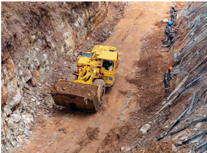
Preparation and rehabilitation of the Qala Adit.
