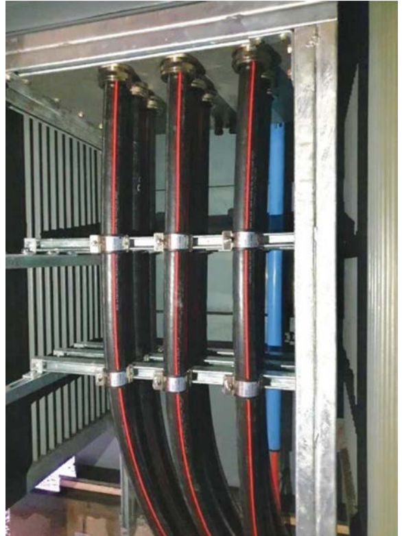
Cleat installation: securing, fixing and routing electrical cables.
