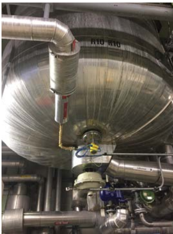
Electronic differential pressure measurement with VEGABAR is silicone oil-free, without capillary lines and requires less installation effort.
