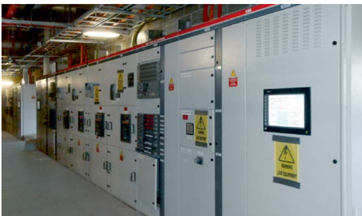
Implementing EtherCAT communications on each generator reduced the wiring requirements and the central control cabinet size to a single 800 mm tier.
