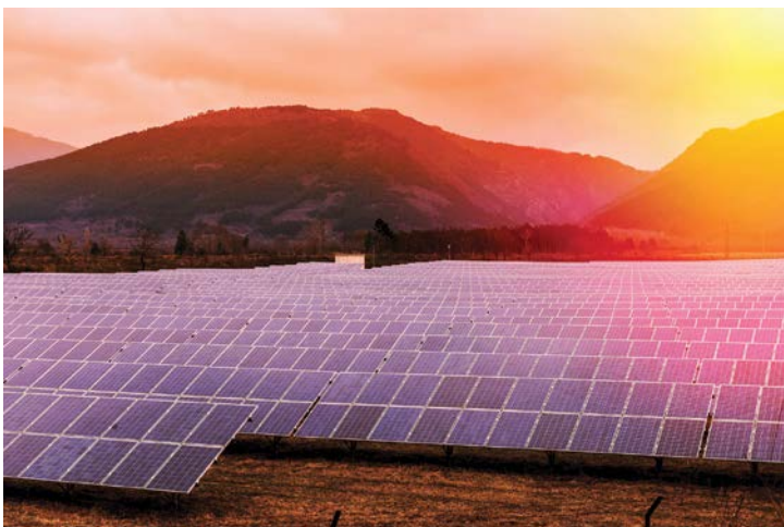
The C&I solar industry is set to see rapid growth and will play a major part in developing the new South African energy mix.
