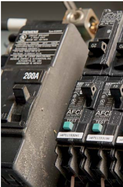
Tools like digital multi-meters and power quality analysers can be used to check and locate power quality problems from the service panel.
