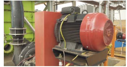
BMG's team of electric motor designers worked with international specialists to develop Synergy IE3 electric motors, setting a benchmark locally for heavy-duty high-efficiency motors.
