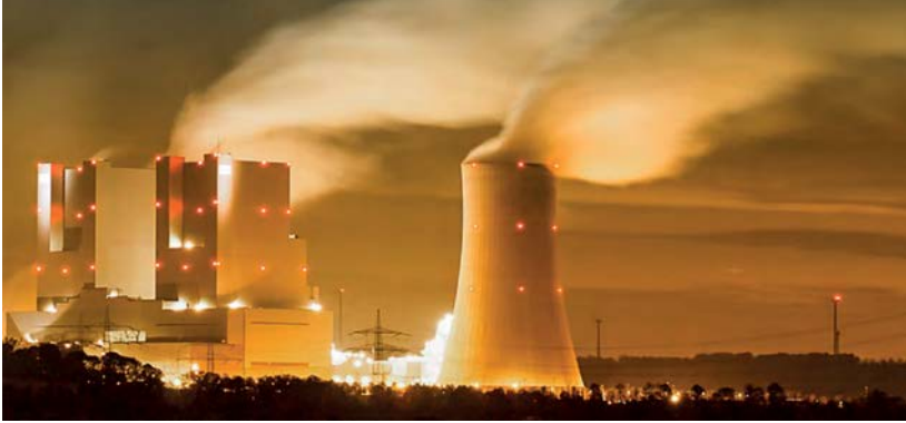
Early detection of boiler tube leaks in power stations has a significant impact in reducing damage and downtime.
