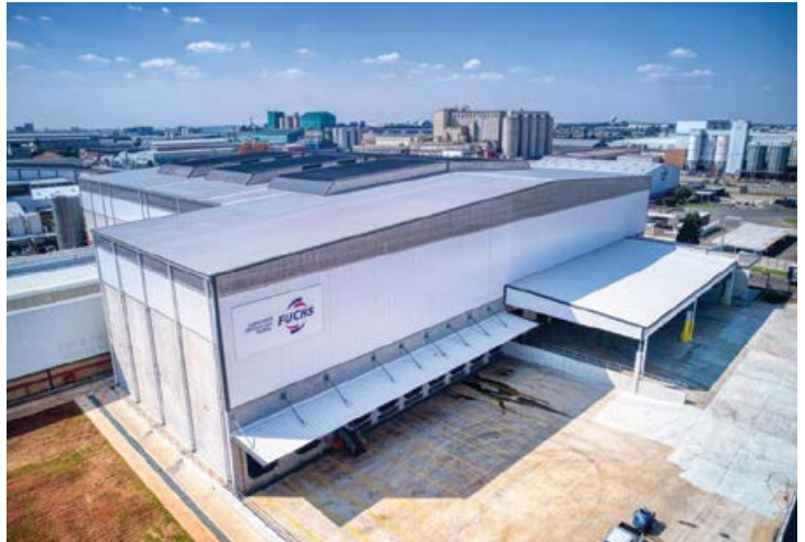
ASP Fire was the fire engineer and ILS the warehouse consultant for the new FUCHS LUBRICANTS South Africa warehouse, a hazardous materials warehouse.
