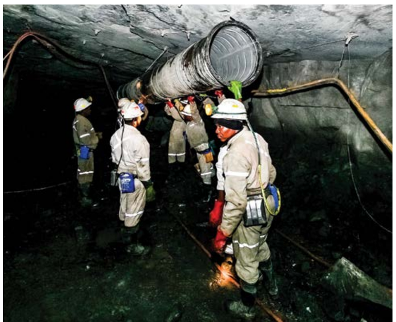
As well as improving efficiencies, a single standard safety induction procedure in mining would support the principle of achieving zero harm.
