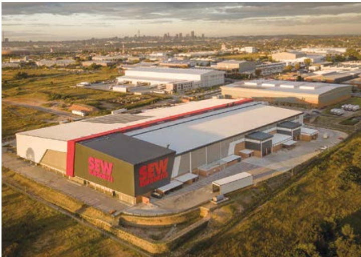
SEW-EURODRIVE South Africa moved into its new 26 000-m 2 headquarters complex south of Johannesburg, in 2022.
