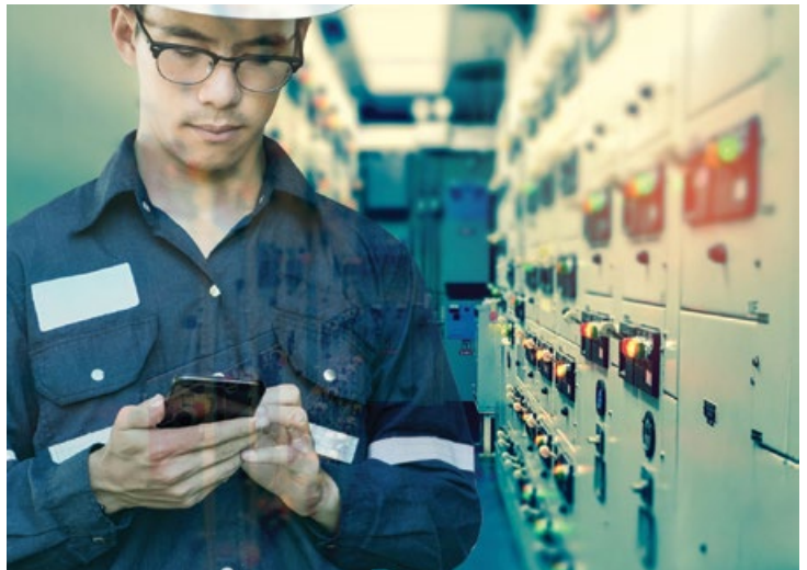
Field services can assist in remotely monitoring connected assets, tracking the health and efficiency of electrical distribution equipment.
