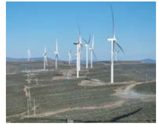
The 147 MW Soetwater wind farm in the Northern Cape is now connected to the electricity grid.
