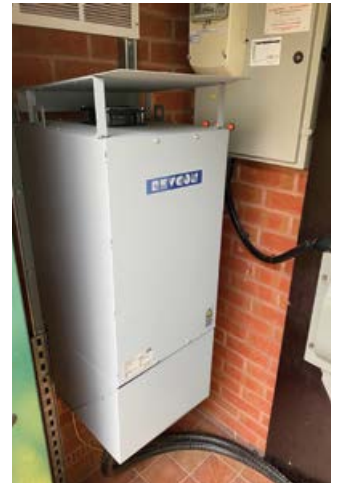
Left: The SineTamer, here installed on a transformer, is a transient voltage surge suppression device. Right: REVCAN Harmonic Filters installed at the high-harmonic sites provide additional protection for the transformer and other nearby equipment.
