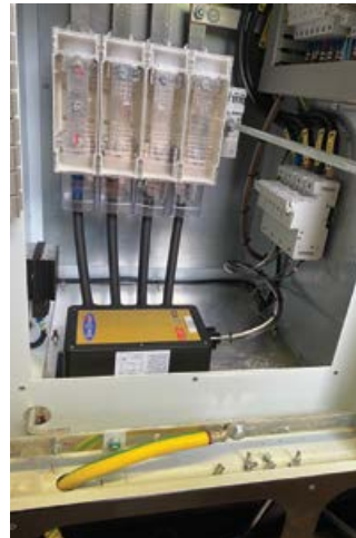
Left: The SineTamer, here installed on a transformer, is a transient voltage surge suppression device. Right: REVCAN Harmonic Filters installed at the high-harmonic sites provide additional protection for the transformer and other nearby equipment.
