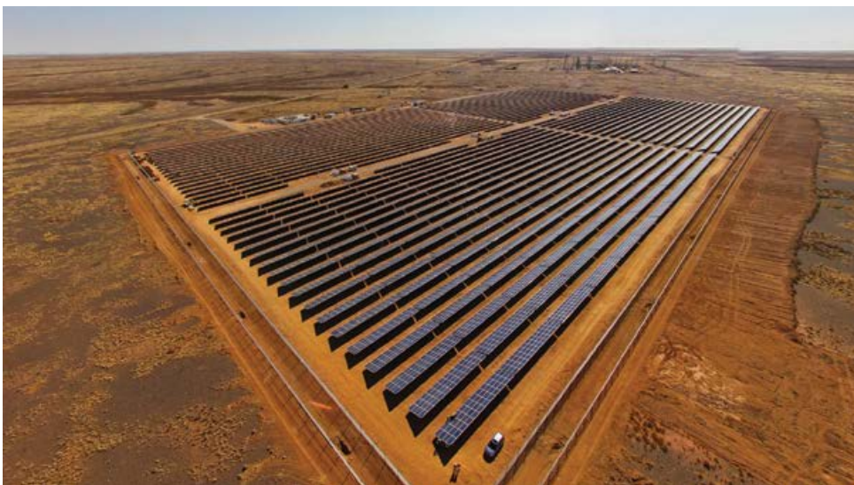
Both the new 100 MW solar PV plants will be 100% South African owned, financed, constructed, operated and managed.
