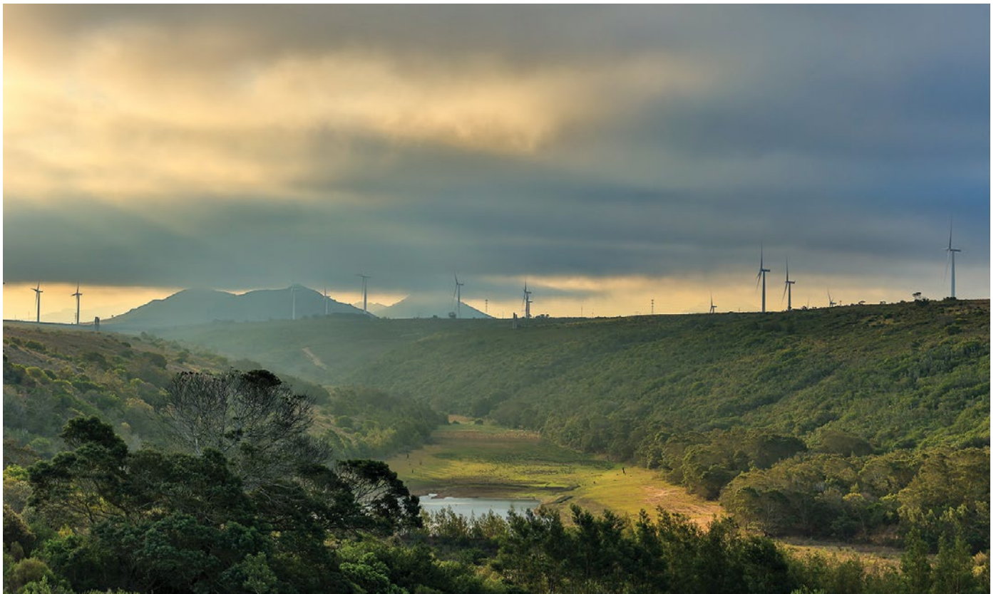
Jeffreys Bay Wind Farm spans 3 700 hectares between Jeffreys Bay and Humansdorp in the Eastern Cape and supplies 460 000 MWh of renewable energy a year to the national grid.
