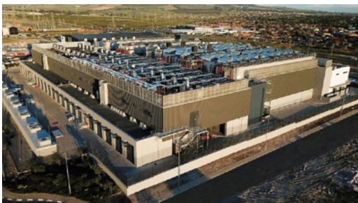
Aerial view of CT2, Teraco's new hyperscale data centre in Brackenfell near Cape Town.
