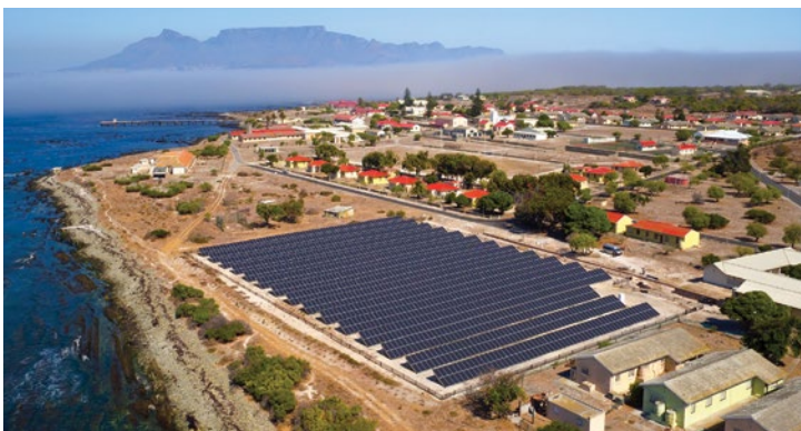
Microgrids and energy storage offer one solution for distributed generation delivering off-grid power supply.
