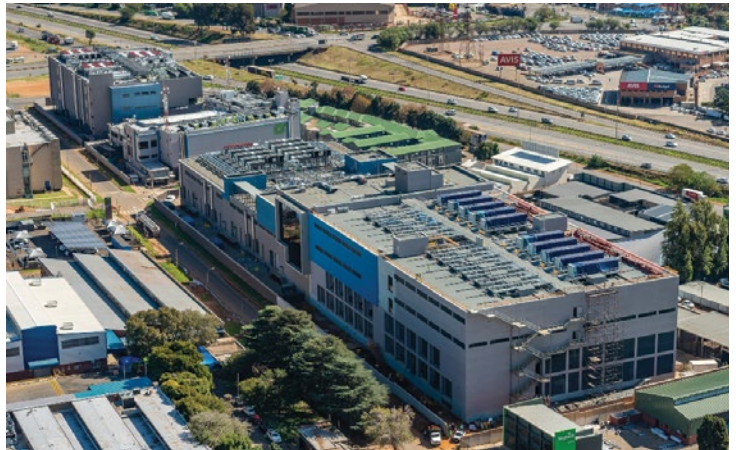
Aerial view of the completed JB3 data centre at Teraco's Isando Campus east of Johannesburg.
