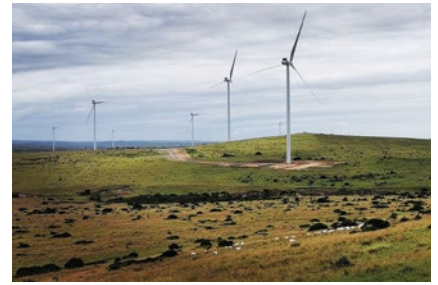
The Wesley-Ciskei wind farm comprises 10 turbines, each with a hub height of 117 m and blades 63 m long.
