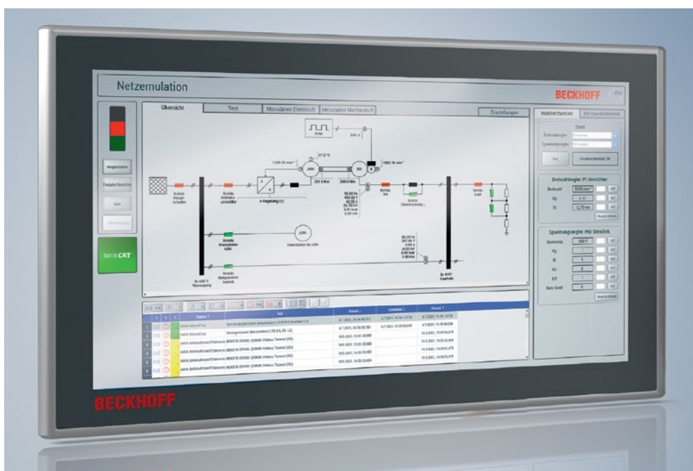
Operation and monitoring of the grid emulation via TwinCAT HMI. © IEH/KIT
