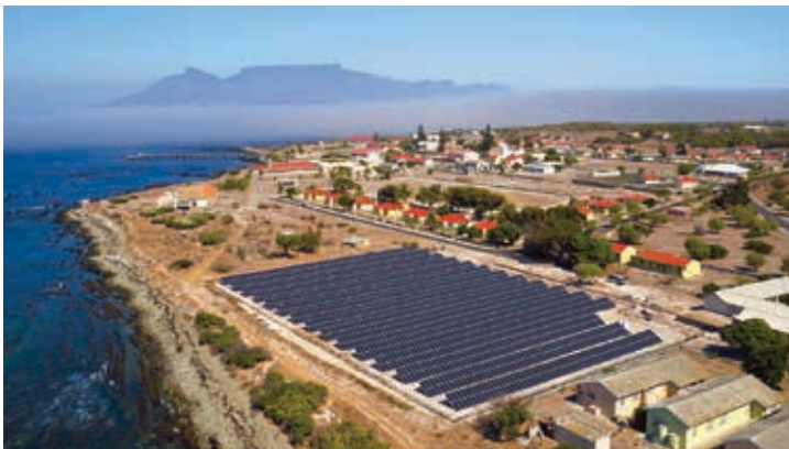
The solar energy powered micro grid with battery bank installed on Robben Island meets all the island's energy needs.
