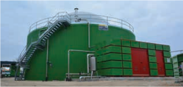
The farm invested in a biomass plant that uses livestock manure and other organic waste to generate energy.
