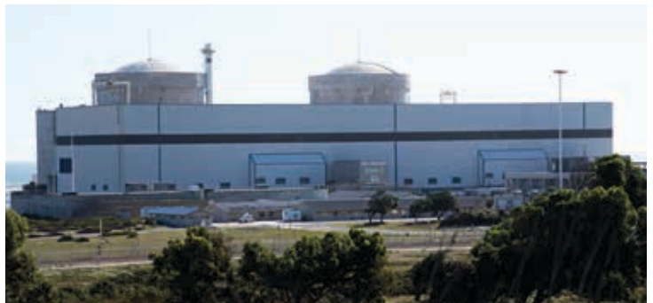
The new replacement steam generators are part of the programme to extend the operating life of Eskom's Koeberg nuclear power station.
