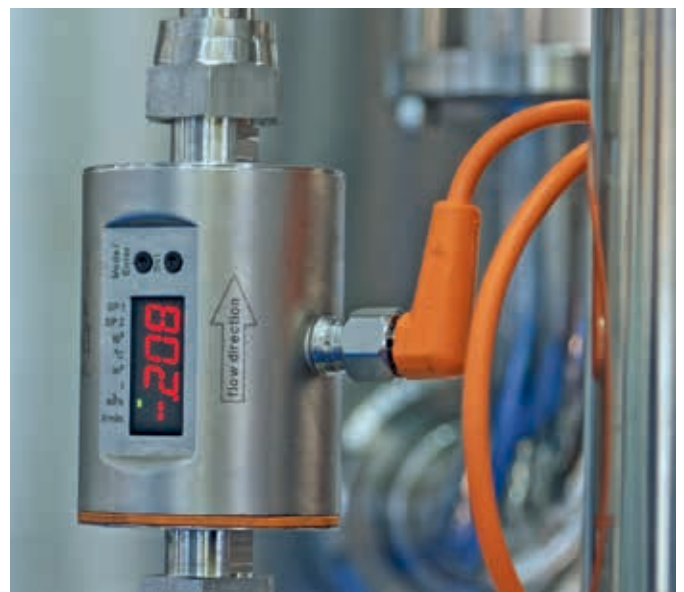
In this HVAC system application the SM6500 magnetic-inductive flow meter delivers high accuracy, repeatability and measurement dynamics to optimise energy efficiency.
