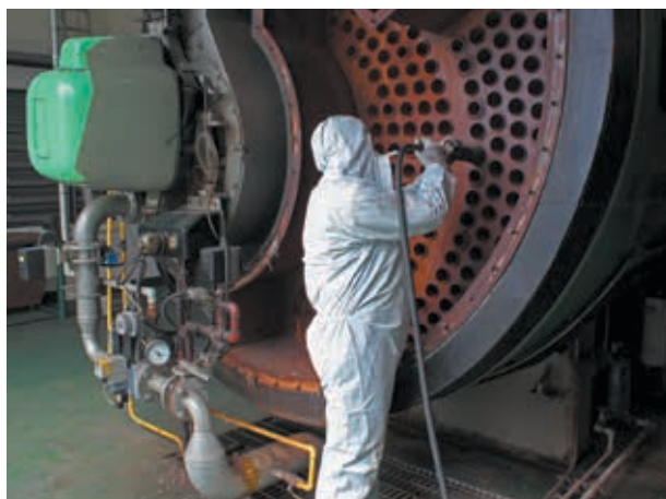
Firetube boilers require regular maintenance to operate at maximum efficiency.
