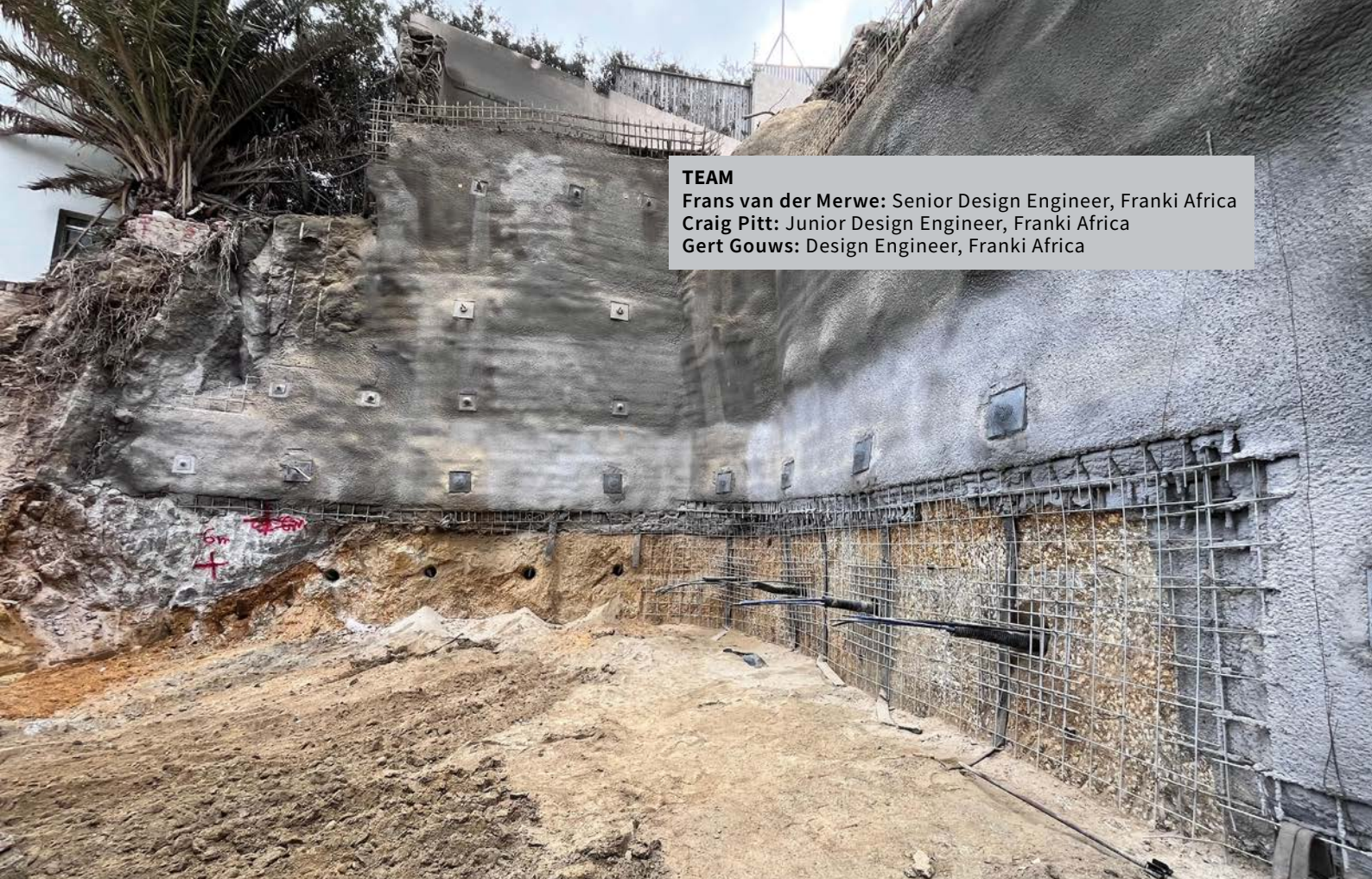
Figure 5: Corestone intercepted in the temporary northern cut face with residual granitic soil below the corestone.
