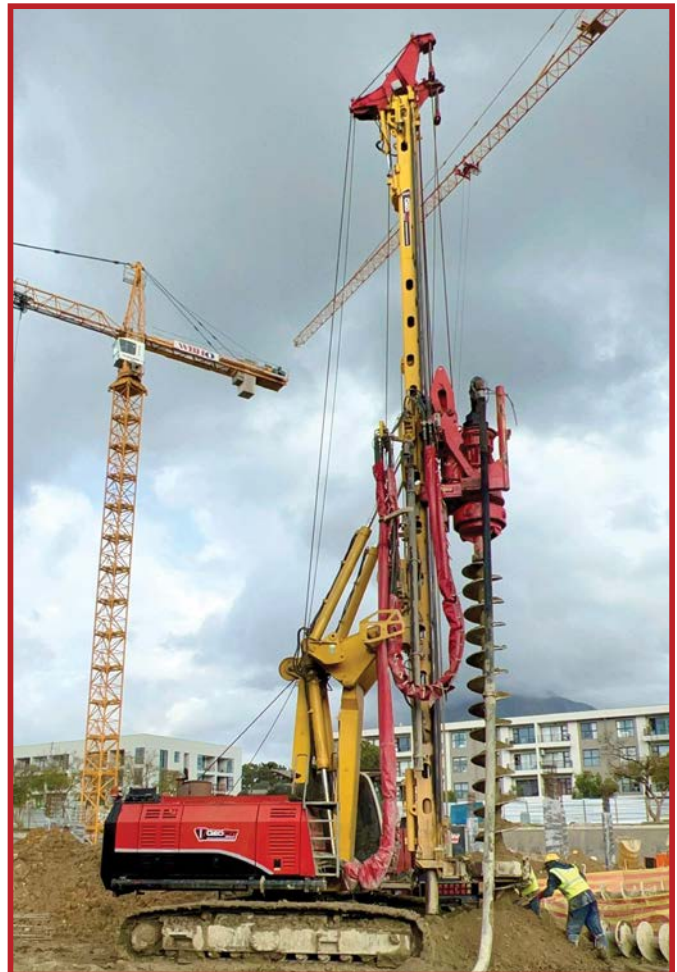
GEOCIV Group's modern fleet of specialised piling and geotechnical equipment.
