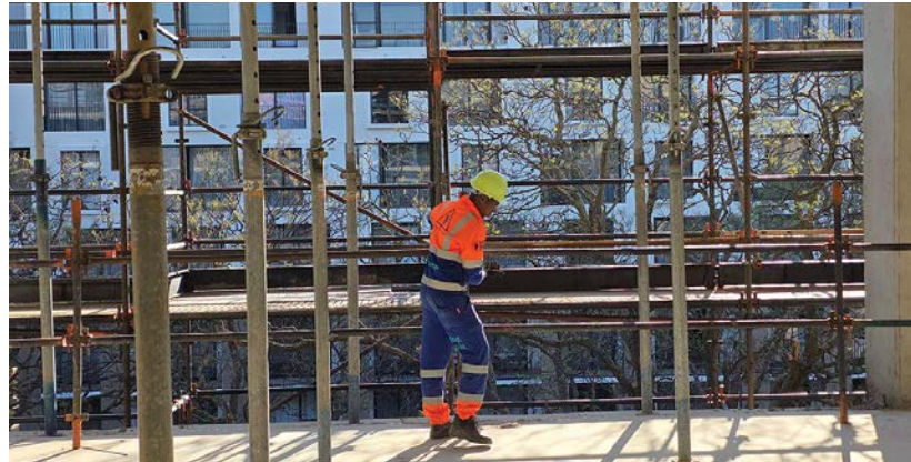
A Concor safety officer inspects slab-edge protection to verify that working-at-height safeguards are properly installed and fully compliant with safety protocols.
