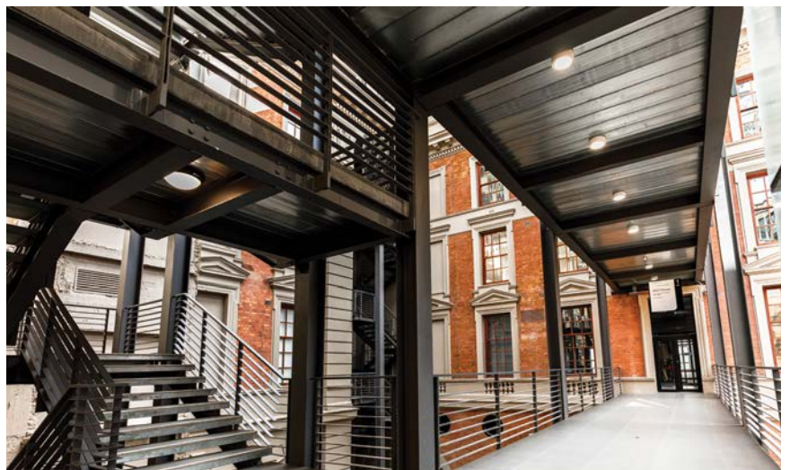
GVK-Siya Zama has officially completed the restoration of 96 Rissik Street in Johannesburg, delivering Transnet's new head office while safeguarding one of the city's most prominent Edwardian landmarks.
