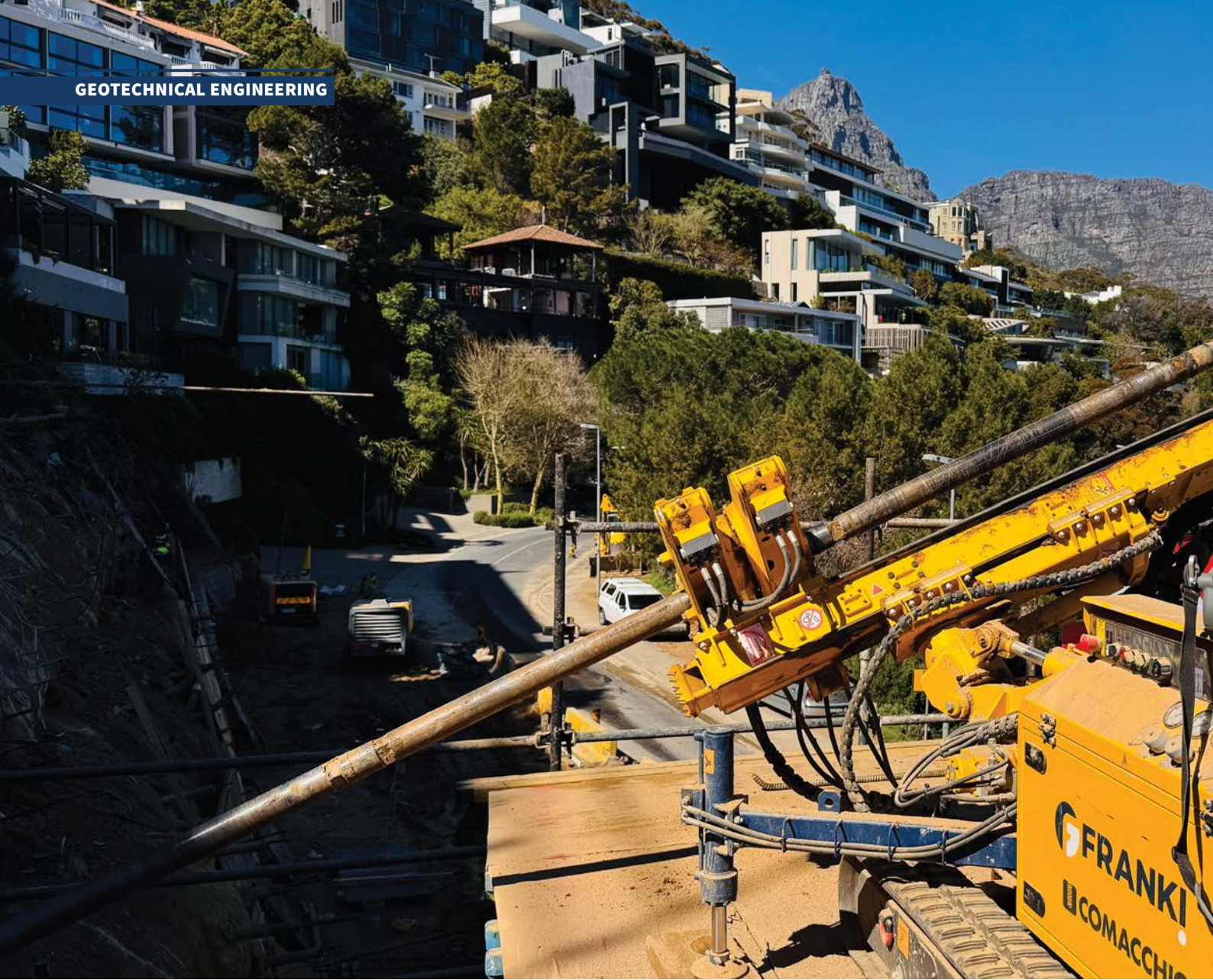
Small rig, big impact! Drilling deep with Franki under mountain views.
