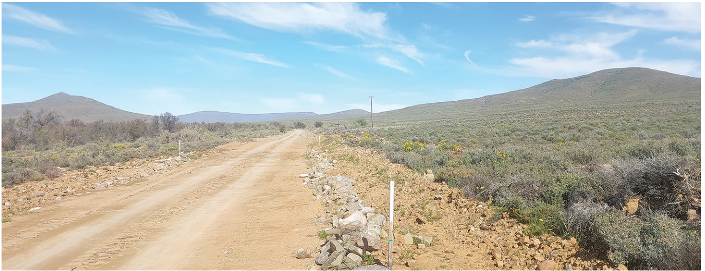
Survey poles demarcate the road servitude at the Karreebosch Wind Farm facility, reinforcing Concor's commitment to sustainable development and environmental stewardship.
