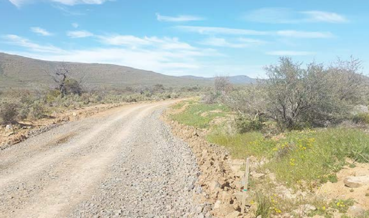
Topsoil is preserved along a road servitude at the Karreebosch Wind Farm facility, ensuring environmental care during construction.
