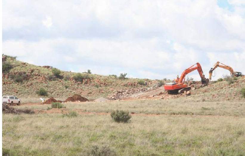
Clearing and grubbing activities underway on the De Aar 2 South Wind Energy Facility project, forming part of the initial site establishment and earthworks phase.
