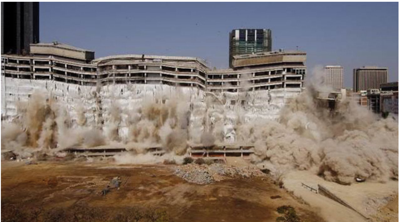
Munitoria Building Implosion.
