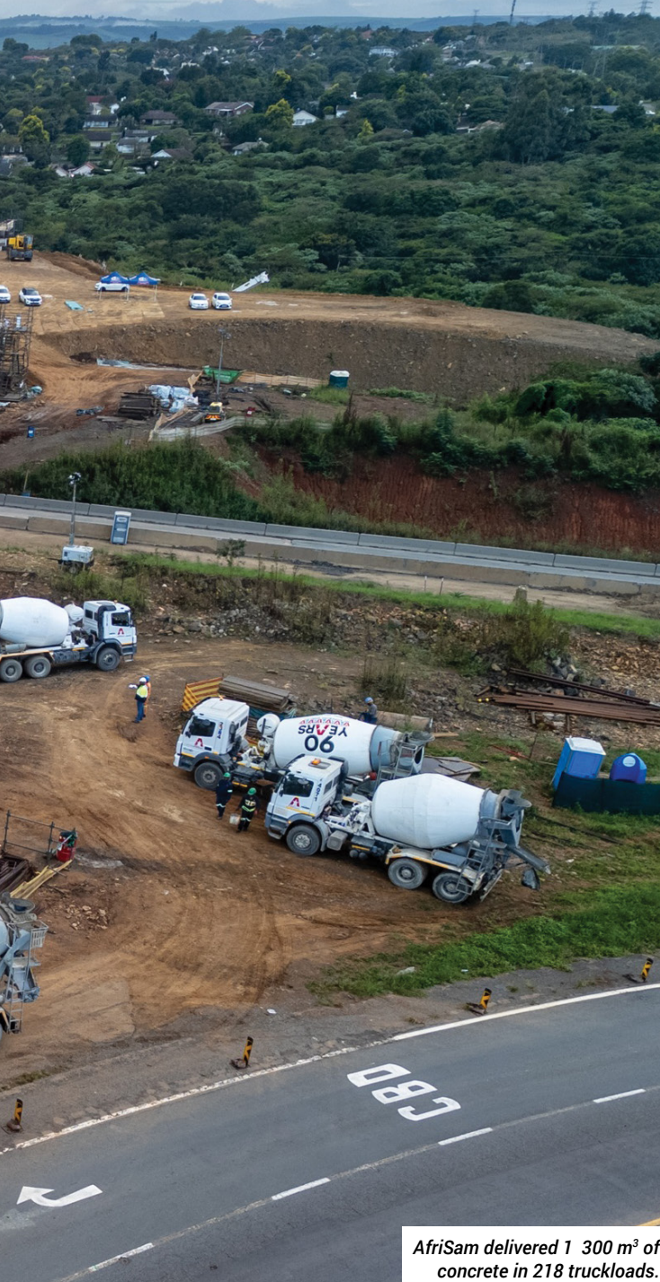
The pour had to be continuous to ensure no cold joints, which meant there was no room for error on this task.
