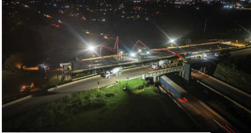
The pour had to be continuous to ensure no cold joints, which meant there was no room for error on this task.
