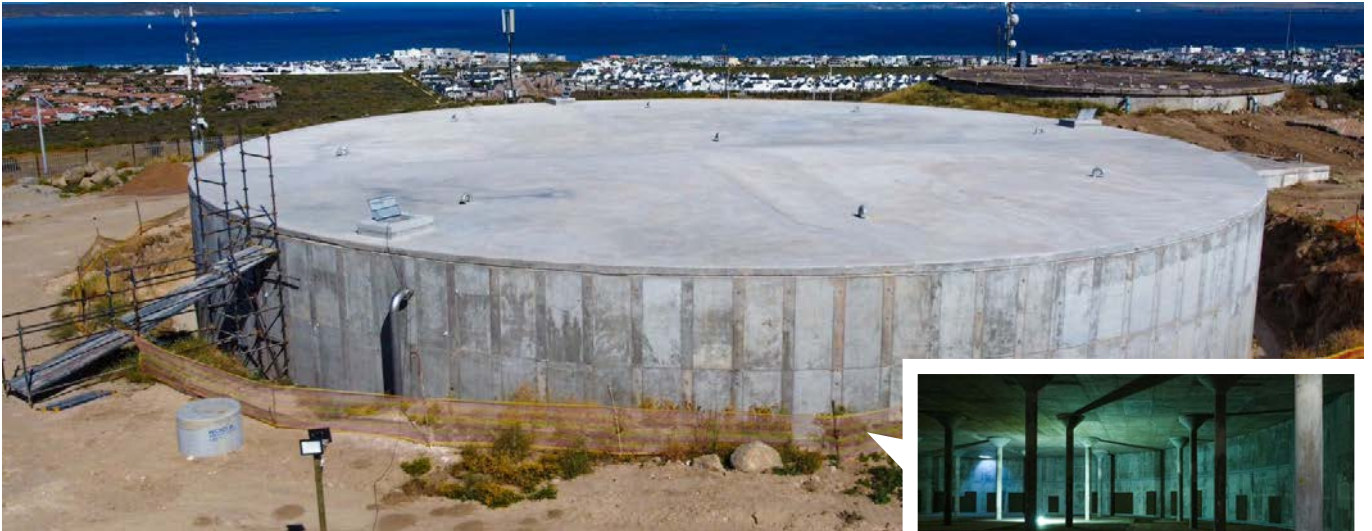
Left: There is no reason that a well designed and built concrete reservoir that is also appropriately maintained should not continue functioning as intended for many years. Right: At 39 m in diameter and 5,5 m deep, the new reservoir was constructed using a conventional reinforced-concrete design.
