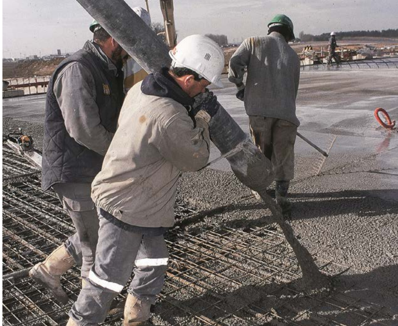
Admixtures ensure smooth concrete flow into tight spaces within steel reinforcement, vital for strength in large water structures.
