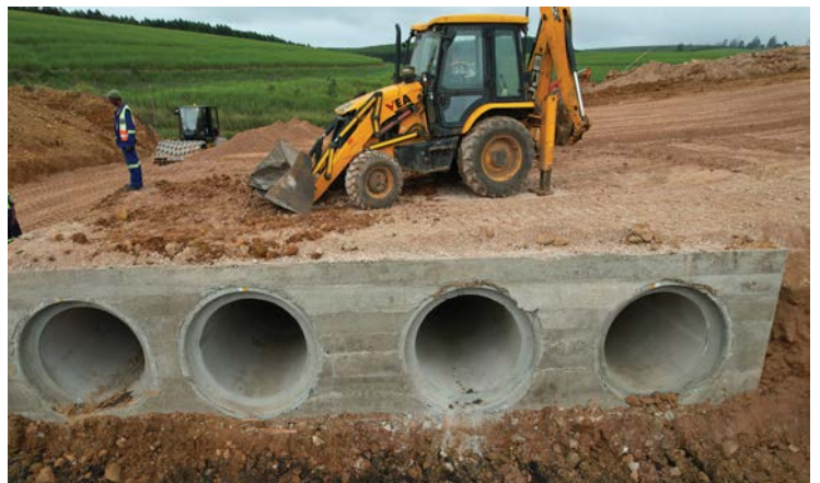
Achieving SANRAL's target date required an all-hands-on-deck approach.
