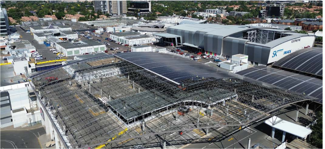
The Eastgate Solar Phase 2 Project won the Innovation and Sustainability Category at this year's Southern Africa Institute of Steel Construction (SAISC) Steel Awards and brought an additional 6,4 MWp of solar power to the iconic Eastgate Shopping Centre in Johannesburg.
