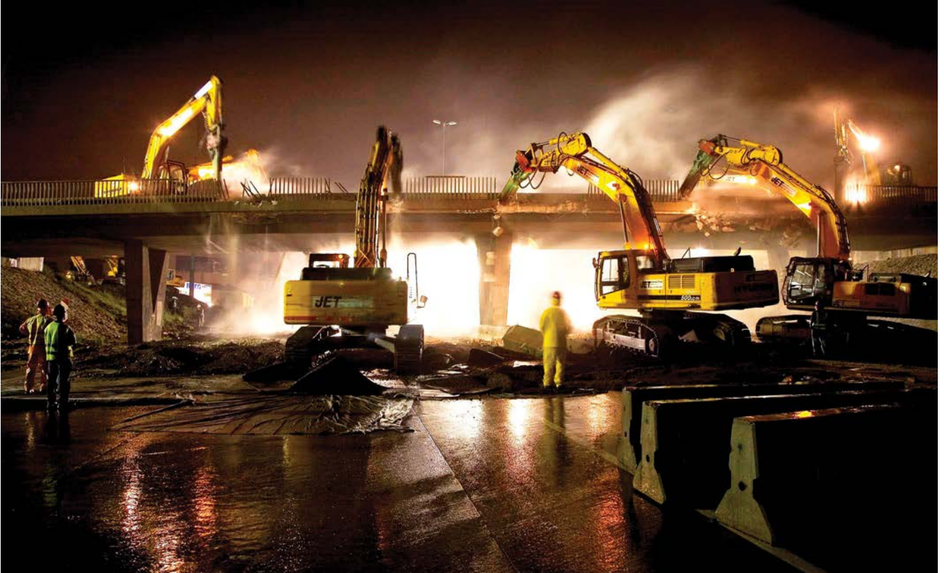
Bridge demolition features increased risk and high-pressure conditions.
