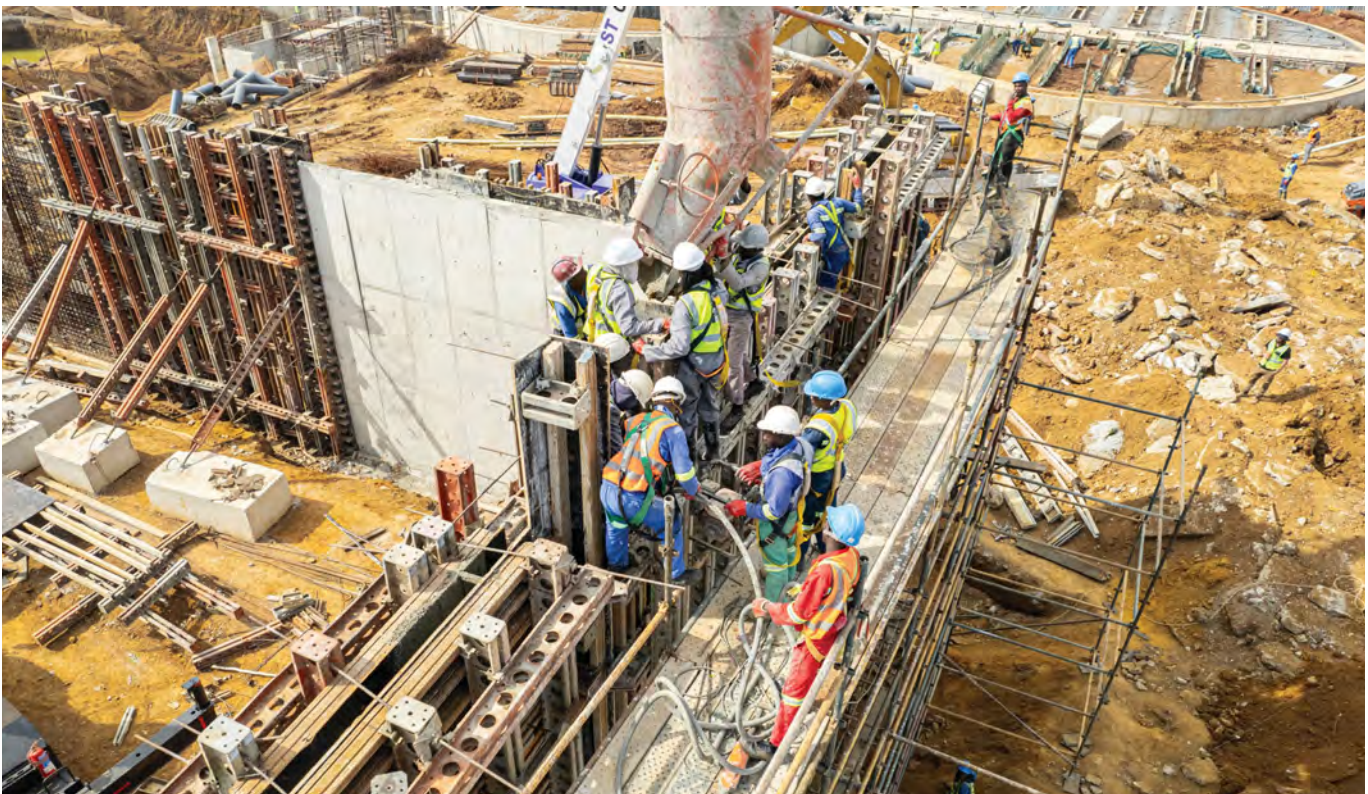
The total concrete volume for constructing the bunker was approximately 1 500 m 3 .
