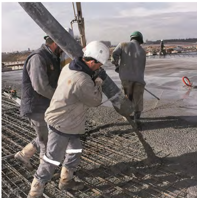
Choosing a non-chloride accelerator is essential when steel reinforcement is present in the concrete.
