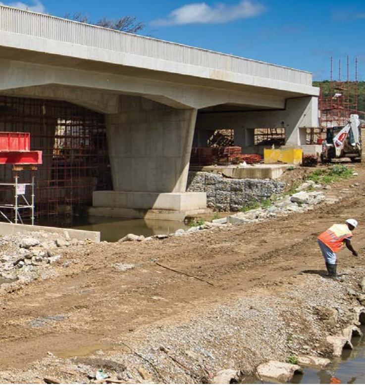
This 140 metre long bridge stands 18 metres above the Tshoxa River and a railway line with a railway bridge, forming a crucial part of a broader road improvement project.
