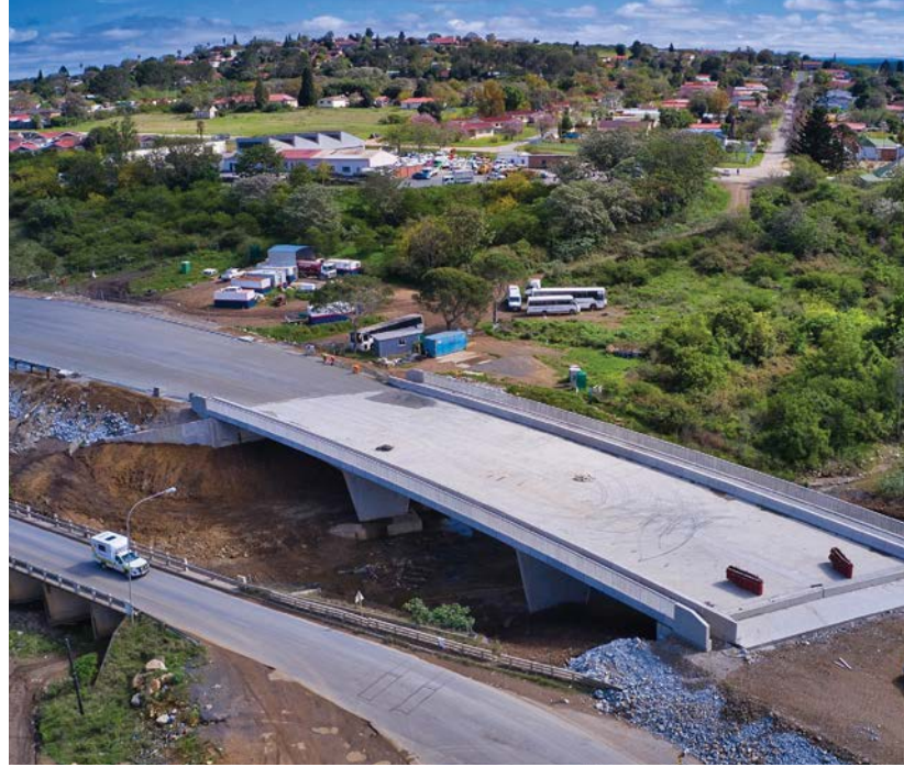
This 140 metre long bridge stands 18 metres above the Tshoxa River and a railway line with a railway bridge, forming a crucial part of a broader road improvement project.
