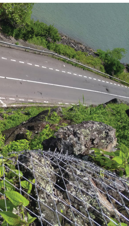
The aim of the Maconde Cliffs project was to stabilise the Maconde cliff over a length of 500 m and to make the B9 road at Maconde safe for road users.
