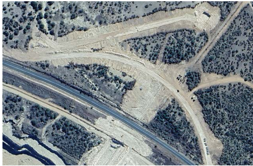
Ulco project area showing the development of the R31 bypass and drainage line diversion above it.
