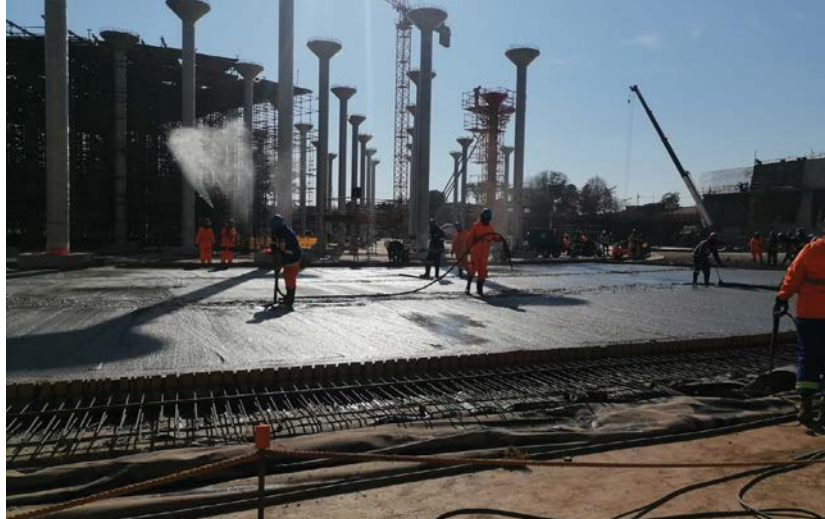
CHRYSO high performance water reducing plasticisers reduce water content, ensuring workability and strength while increasing the slump.
