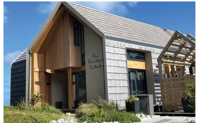
Left: One of the Western Cape’s most-loved concrete roof tiles, Eagle Roof Tile’s Shingle profile lends itself to the sharp triangular lines on this exposed intersecting gable roof. Right: Eagle Roof Tile’s slate grey shingle as seen on this A-frame with exposed gables in Eerste Rivier, Western Cape, was used to cover the roof and clad the vertical sides.
