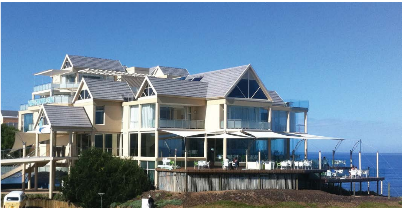
Covered with Eagle Roof Tile’s slate tile, modern elegance gives way to crisscrossing angles and framed gables at The Waves in Wilderness, Western Cape.
