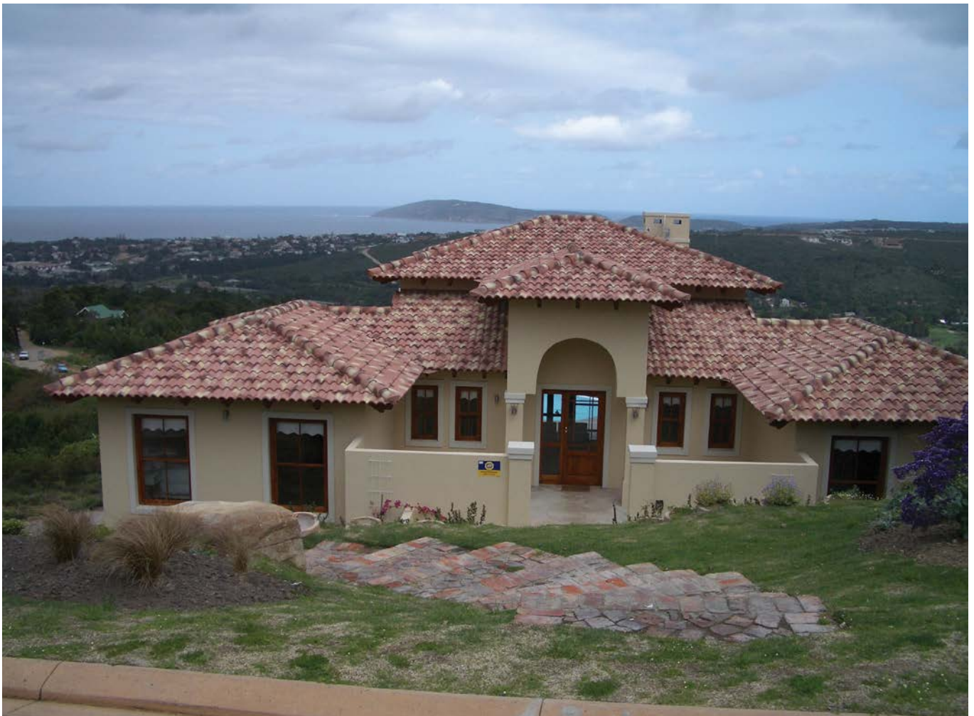
A Plettenberg Bay house where Eagle Roof Tile's Tuscan profile tile was used on this Spanish-inspired hip-roof with exposed eaves and verges.
