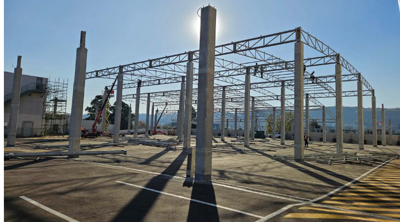
Erection of the steel framework structure underway on one section.
