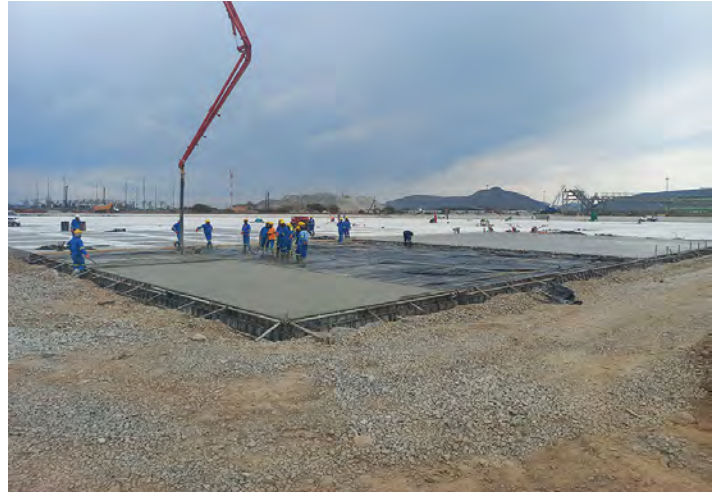
Concrete slabs for the Merensky stock pad at Bakubung Platinum.
