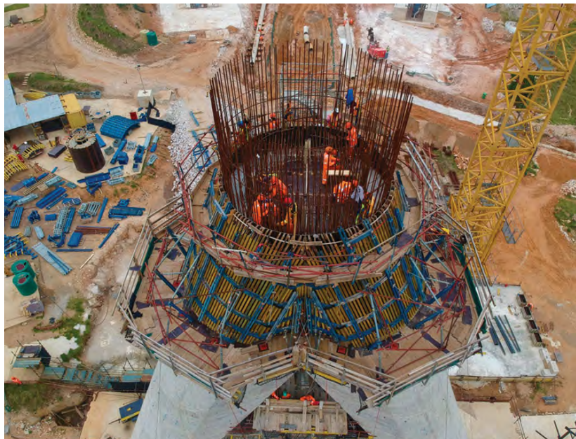
Steel fixing of the bifurcation lift soffit slab in October 2022.
