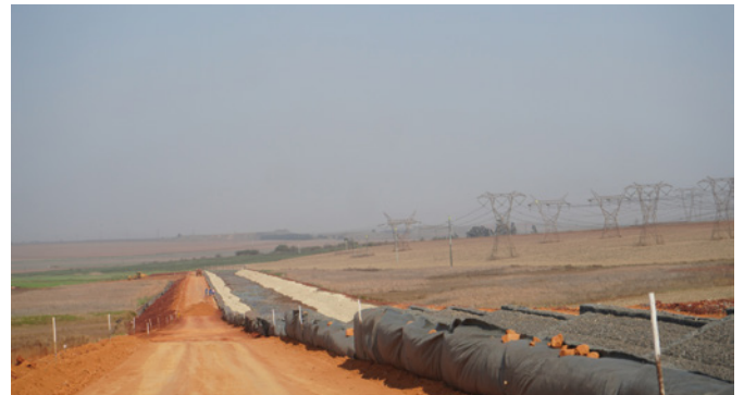
The stream diversion will channel clean water around the ADF area.
