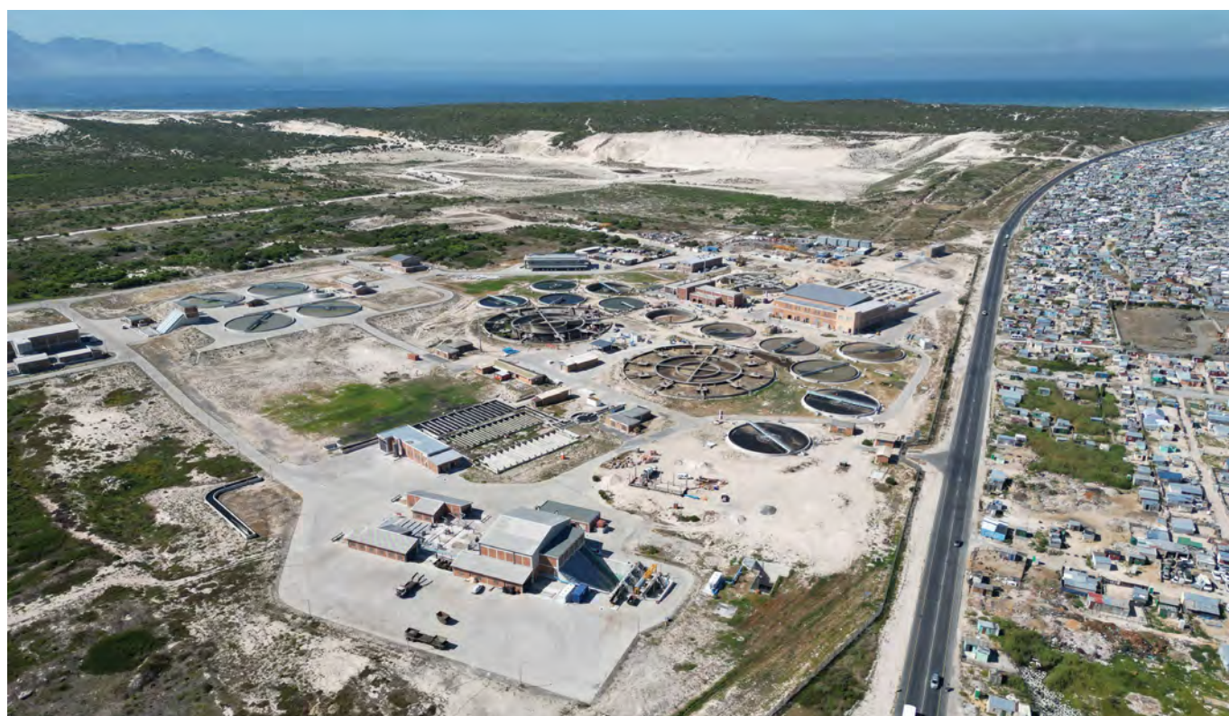
Zandvliet Wastewater WWTW is the third largest in Cape Town.
