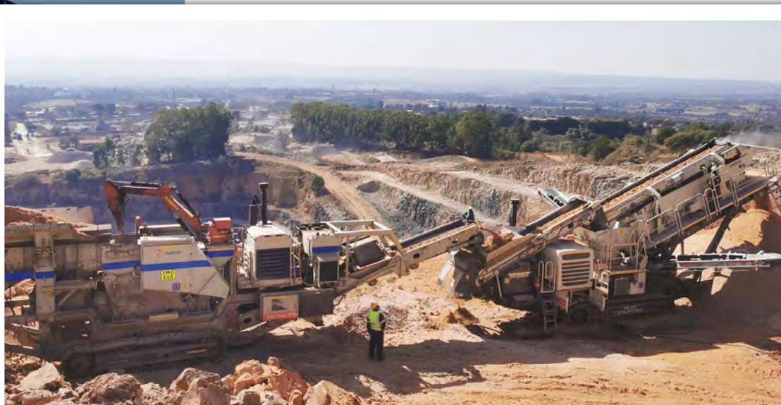
Metso LT110 and LT220D mobiles crushing aggregates in a quarry.
