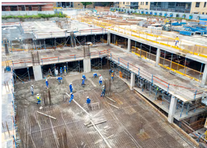
Readymix concrete is pumped for the in-situ construction of post-tension slabs.
