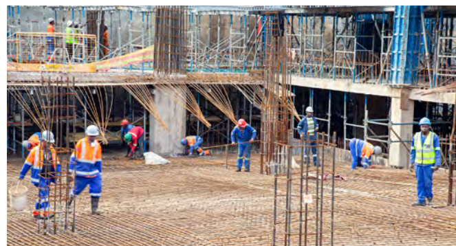
Left: Concor is currently building a super-basement as the first phase of the Trevenna Office Campus. Right: The structure will contain 2 300 tons of rebar.
