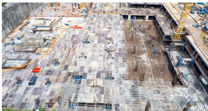
Left: Concor is currently building a super-basement as the first phase of the Trevenna Office Campus. Right: The structure will contain 2 300 tons of rebar.
