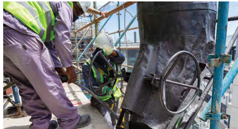
About 10 different concrete mixes were employed during the project to suit various applications.
