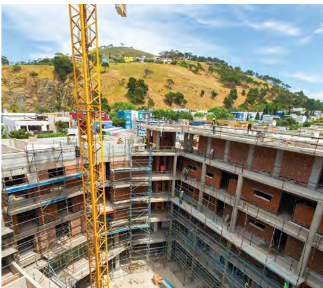
Left: The project is adding four floors of luxury apartments onto the existing retail level, with three basements. Right: A particular challenge was the lack of space in the basement for the use of normal Class 3 formwork.
