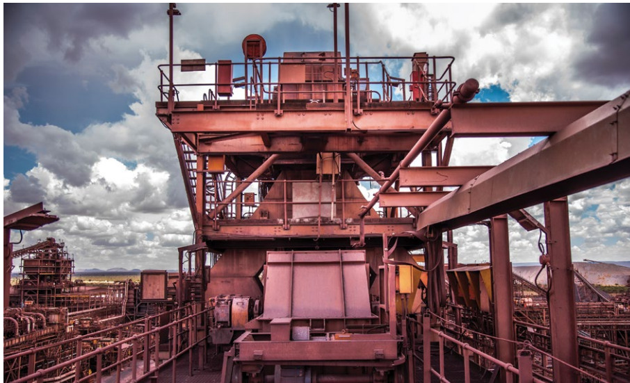
The feed conveyor discharge chute at an iron ore mine is designed for seamless material transfer, reducing spillage and dust while improving efficiency.
