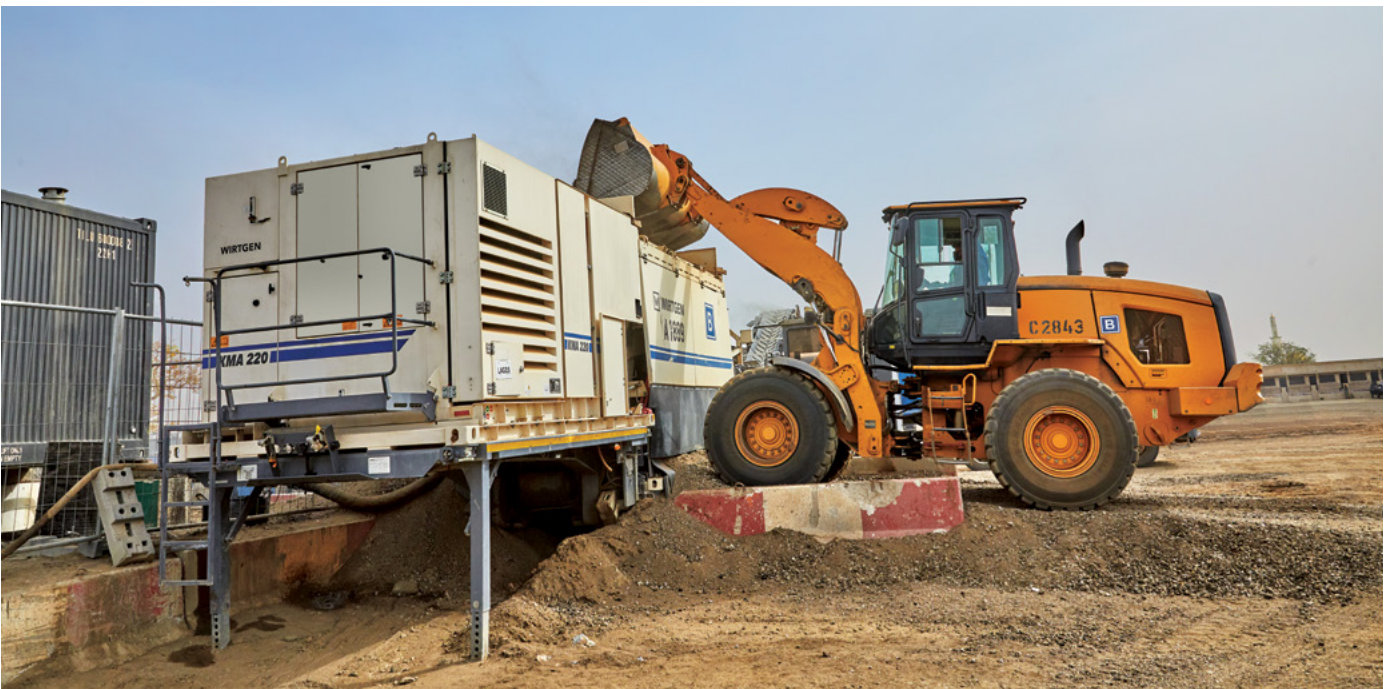
Wheel loaders feed the crushed material to the Wirtgen KMA 220.
