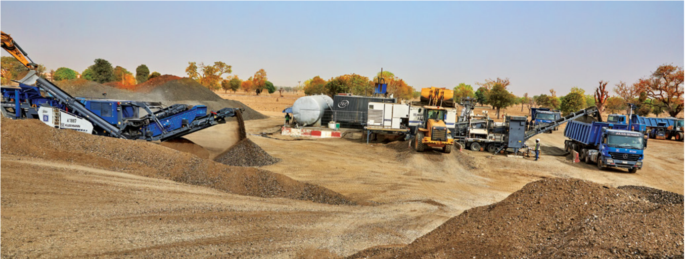
An ideally coordinated team: the Kleemann MOBIREX MR 110Z EVO2 impact crusher reduces the milled material to the required grain size. Parallel to this, the KMA 220 processes crushed milled material to a new mix and loads it directly onto trucks.
