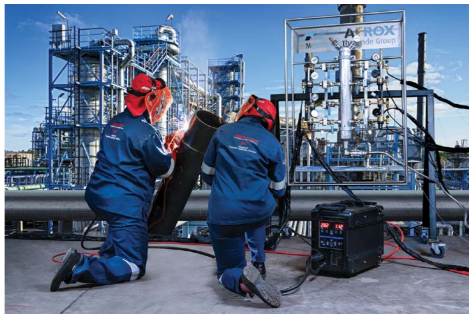
ArcReach™ technology removes the need for transporting welding machines up and down a construction site, and if used together with GasReach, completely eliminates the associated logistics and safety nightmare.
