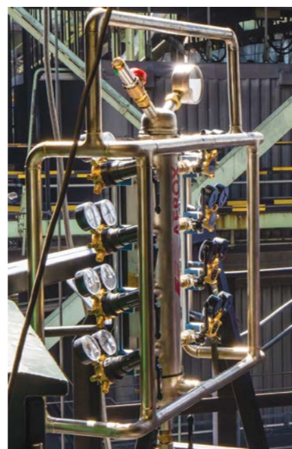
With GasReach, a multi-user pressure panel (MUPP) is installed at hard-to-reach welding locations to completely overcome the problem of transporting full and empty gas cylinders to and from the working area.
