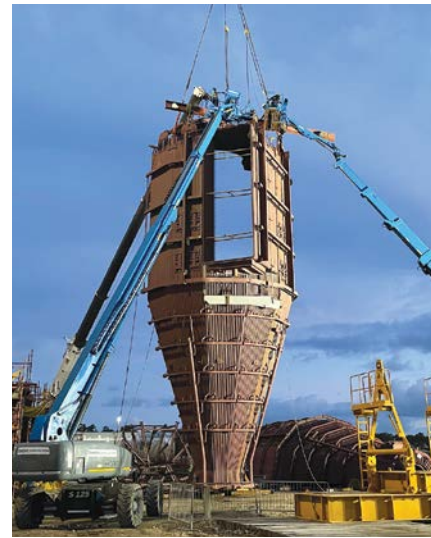
A pre-fabricated conical section being installed in the Mondi boiler.
