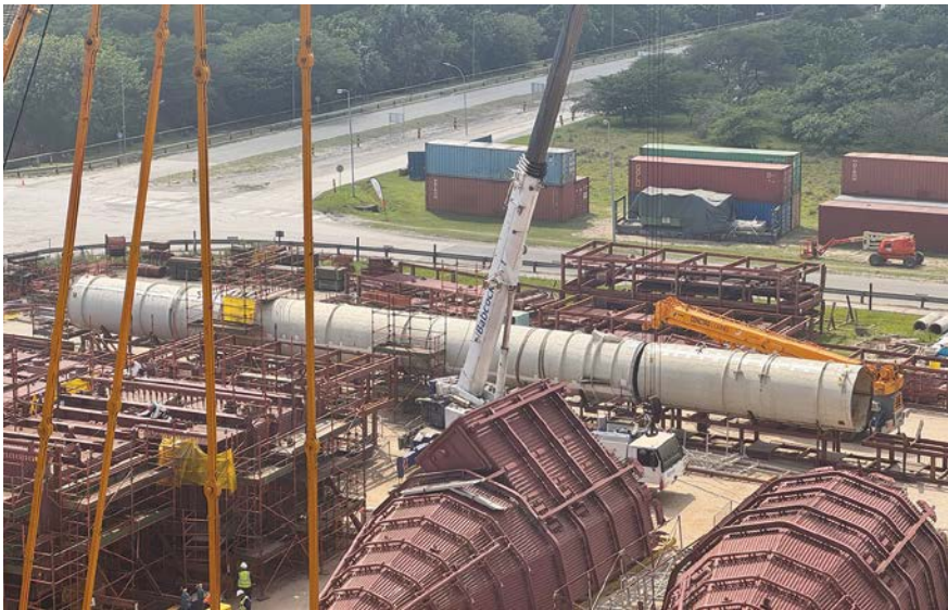
A flue gas stack is being prefabricated at the construction site.
