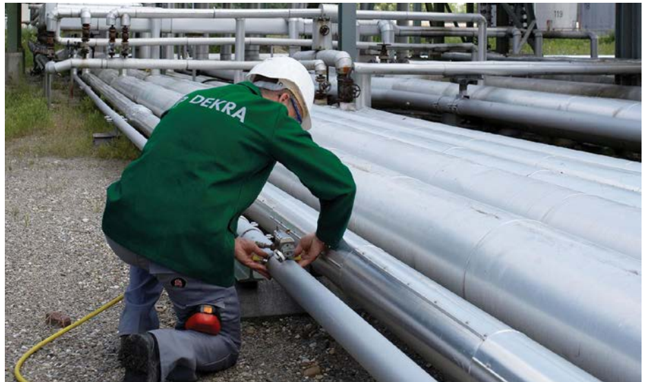
A DEKRA NDT Inspector performs radiographic testing (RT) of butt welds using Gamma radiation.
