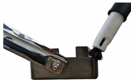
A current-conducting carbon fibre brush is used to apply the solution to any discoloured areas of the stainless steel, which both removes the damaged surface oxides and passivates the chromium-rich surface layer at the same time.
