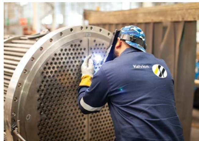
Most of the heat exchanger and waste heat boiler work done at Kelvion's facility in Roodekop requires high integrity fusion welds between the tubes and the tubesheet.
